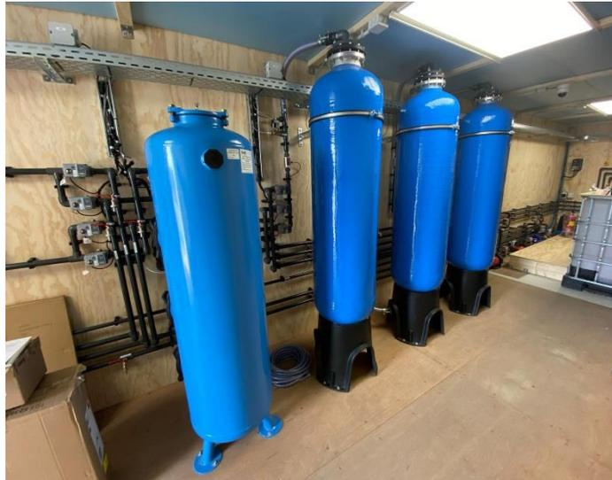
Figure 27. BioPhree filter and adsorption columns
