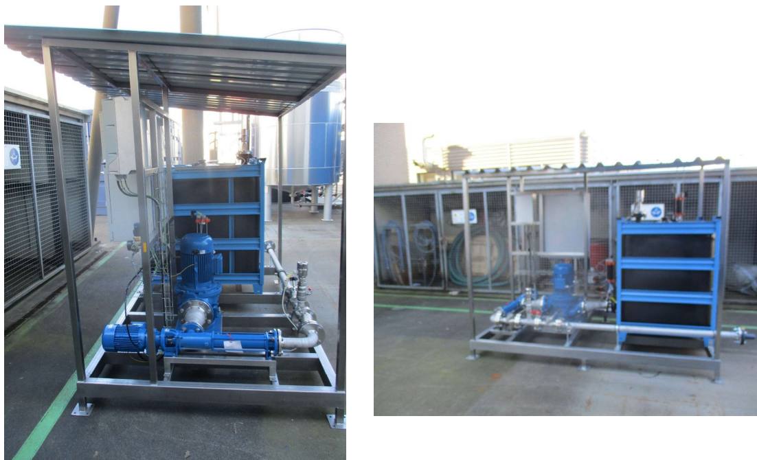
Figure 4:. The feed skid with a 1000 L feed buffer tank, a macerator and cavity pump.
