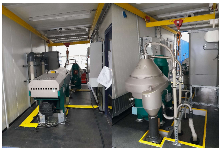
Figure 12: Decanter centrifuge (left) and disc centrifuge –a.k.a. separator (right).
