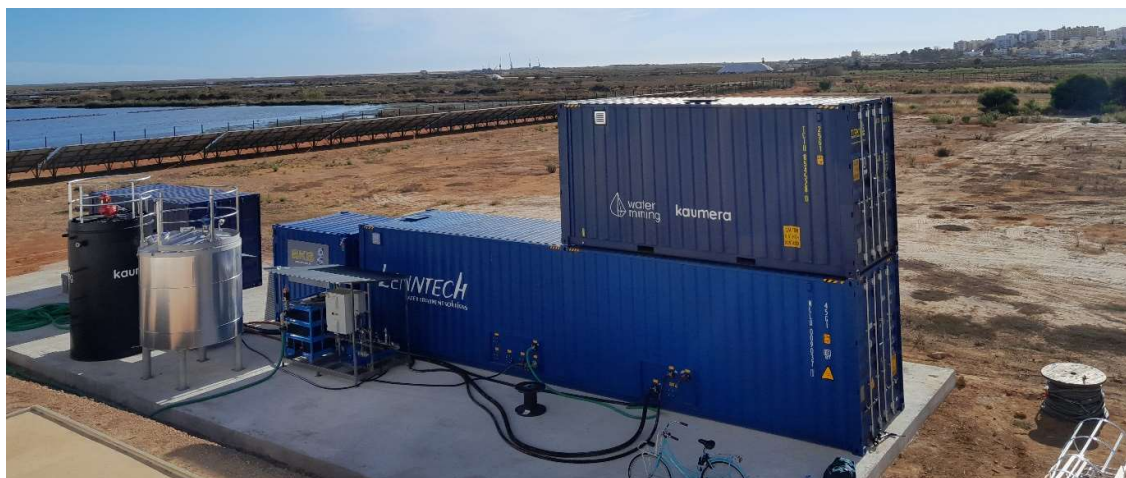
Figure 16: Assembly of the pilot installation in Faro/Olhão in progress.
