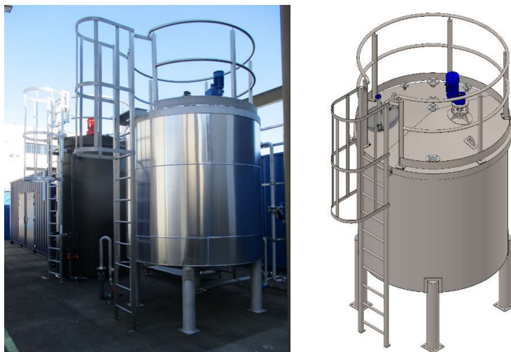
Figure 5: The reactor tank for alkalinsation and heating up the excess sludge.
